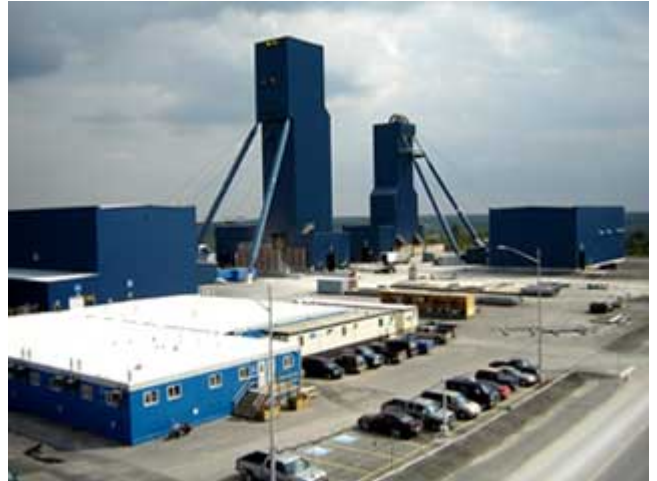
Falconbridge Ltd. is investing $514 million in its new Nickel Rim South mine project in Sudbury.
